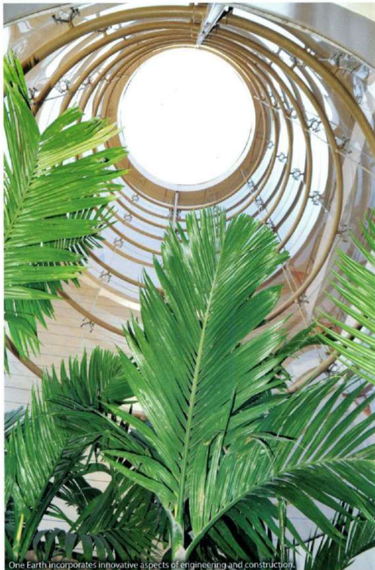
One Earth incorporates innovative aspects of engineering and construction.
