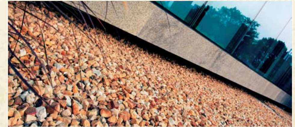
The pebble drain from where all excess water on hard surfaces is drained out
