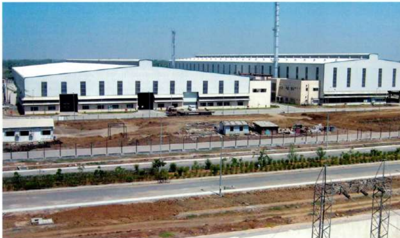
■ The SE forge premises at the industrial park in Vadodara.
